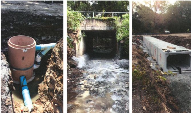
53rd Street Utility Relocation
