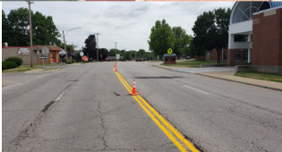
Pavement Marking Project
